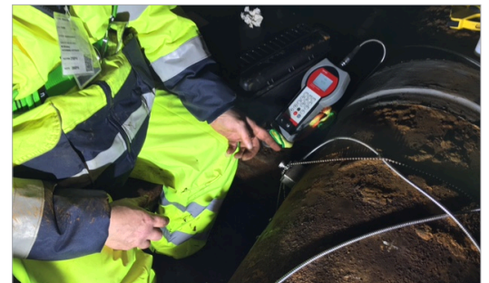
A KATflow 200 portable flowmeter was used to survey the pipe prior to full installation
