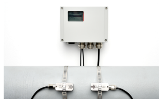
Two KATflow 100 flowmeters were installed as part of a permanent metering and monitoring package.
